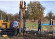
深水井施工 Deep well construction
