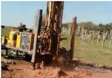
深水井施工 Deep well construction
